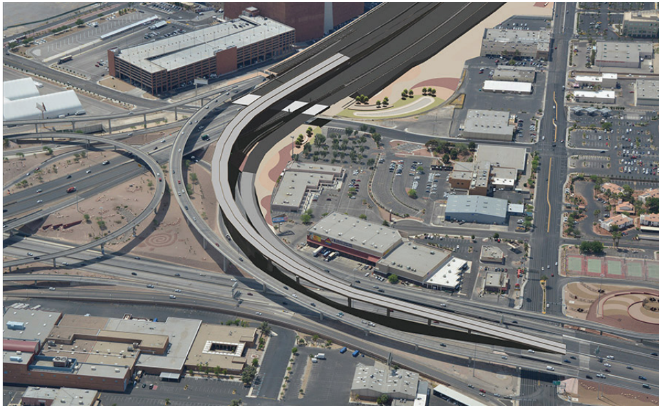
Winning bid beats runners up on cost and time for the 3.7 mile I-15 widening project that includes the downtown "spaghetti bowl" interchange
